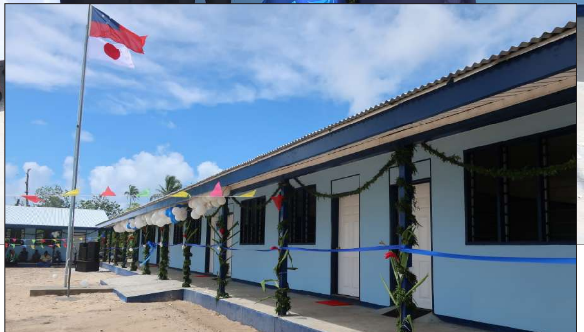
The new school building of Faga Primary School successfully funded under Japan's GGP
