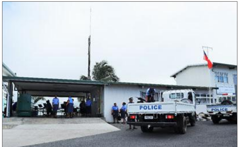
The look of the new upgrade and renovation works to the Maritime Wing of the Samoa Police. Photo: Tusiga Taofiga.
