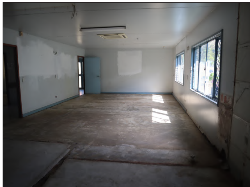
Inside the old MEDCEN hospital
