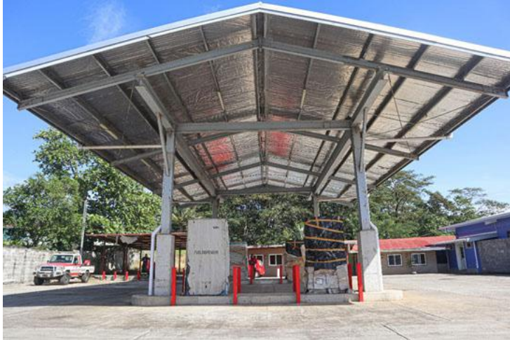
The Petrol Station at Tuana'imato across from the Fire Station designated for the transport refuel and car park for all vehicles for C.H.O.G.M. 2024. Photo: Leota Marc Membrere
