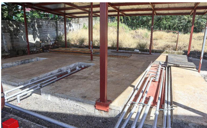
Tank Shelter. Photo: Leota Marc Membrere
